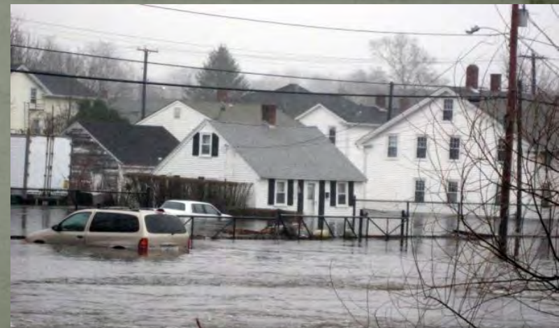
Moderate flooding along Connecticut River, April 1 st , 2010. Photo: NBC Connecticut
